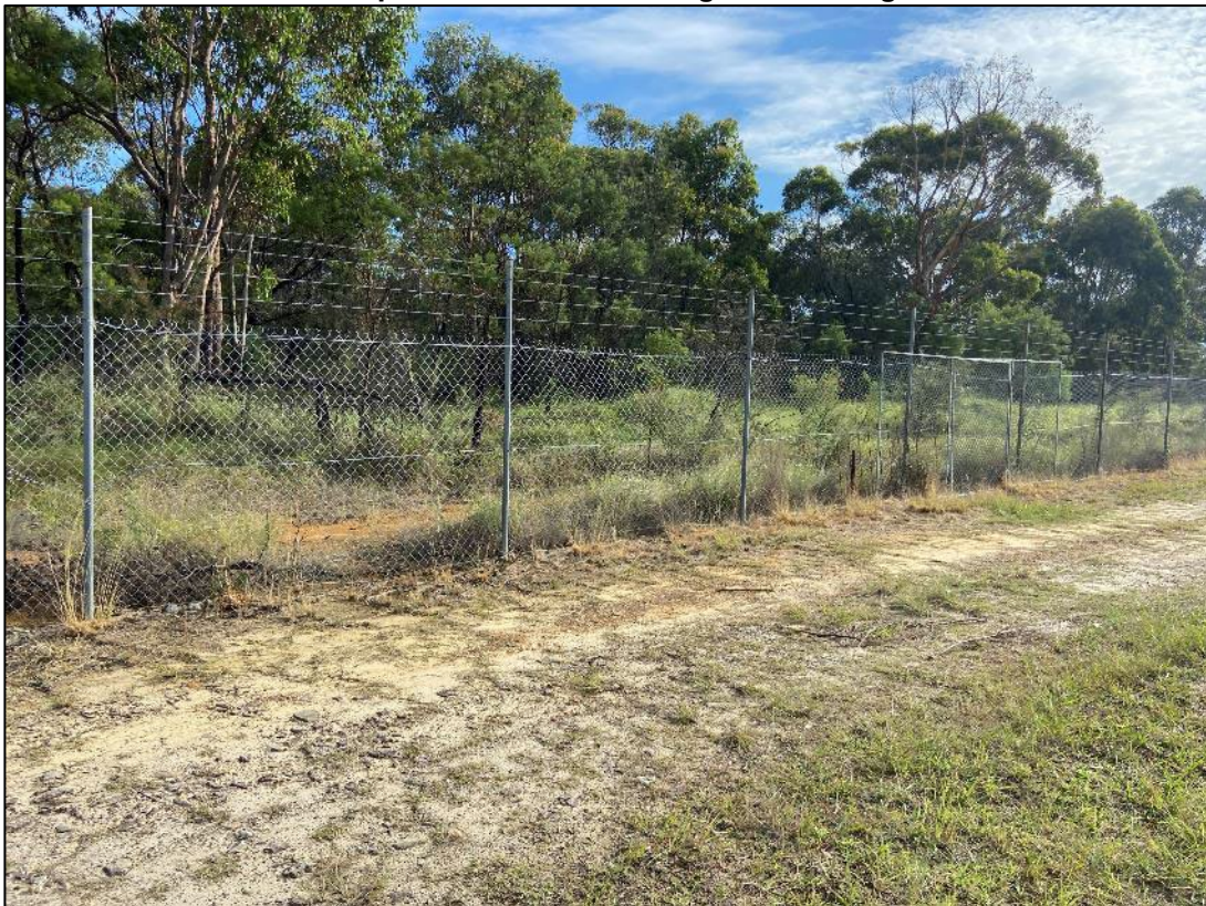
Below: Example of chain-link fencing surrounding the site.
